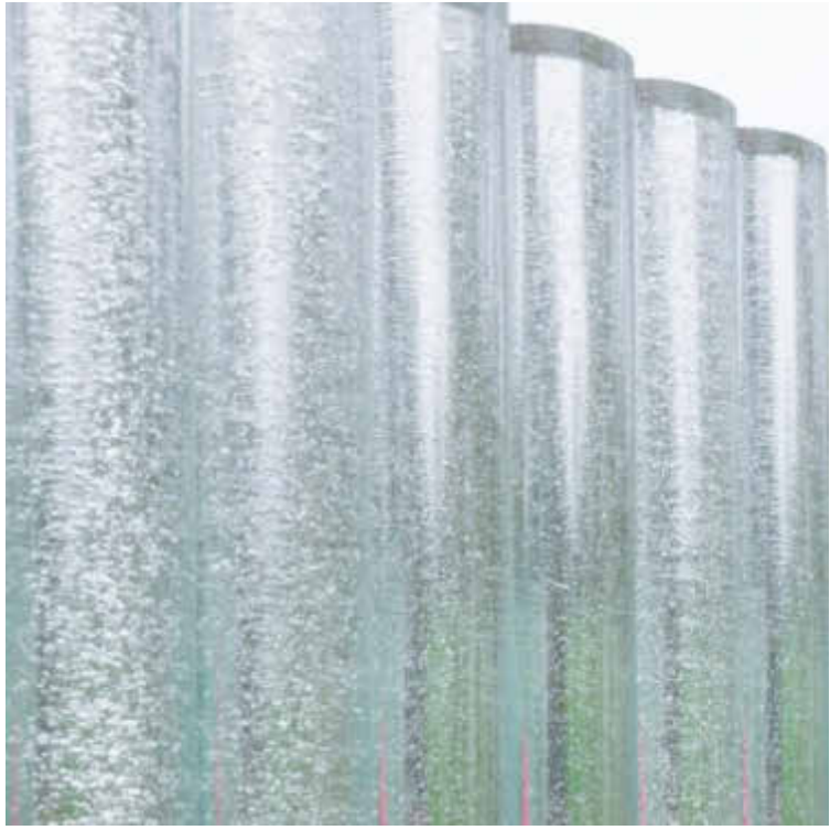
GB 02 GLASS COLUMNS STACKED CAST GLASS BLOCKS ON ANCHOR RODS WITH LED LIGHTING BEHIND
